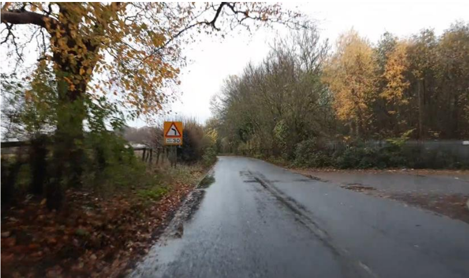
Existing road narrows warning signage for eastbound traffic on C234 at Hardhaugh
